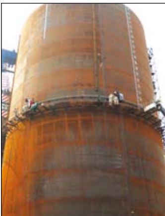
AGWI/P for tower welding
