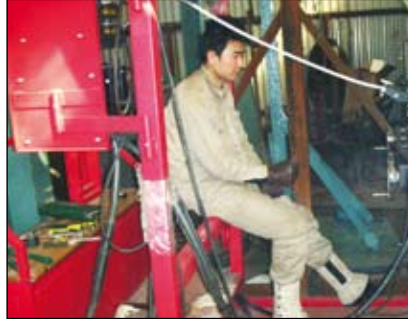
All Time girth welder with expandable base for welding the cone segment of a blast furnace
