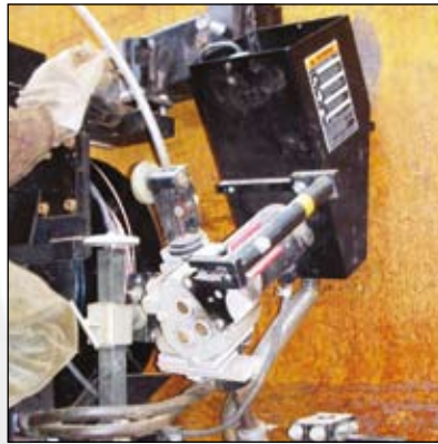
Tank base plate OD fillet welding
