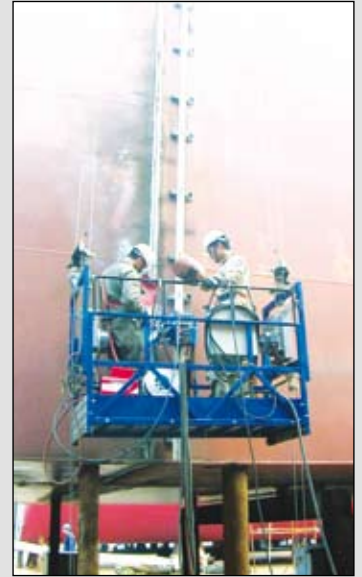
EGW carriage to be used with standard gondola for ship panel vertical welding
