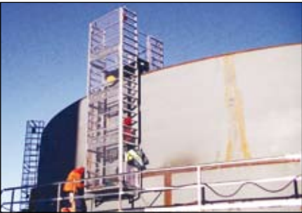
Meshed frame for safe operation on site
