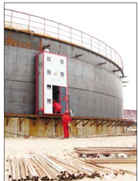
EGWI/D travels on based mounted rail for top down tank erection
