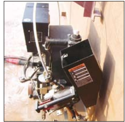
Tank base plate ID fillet welding
